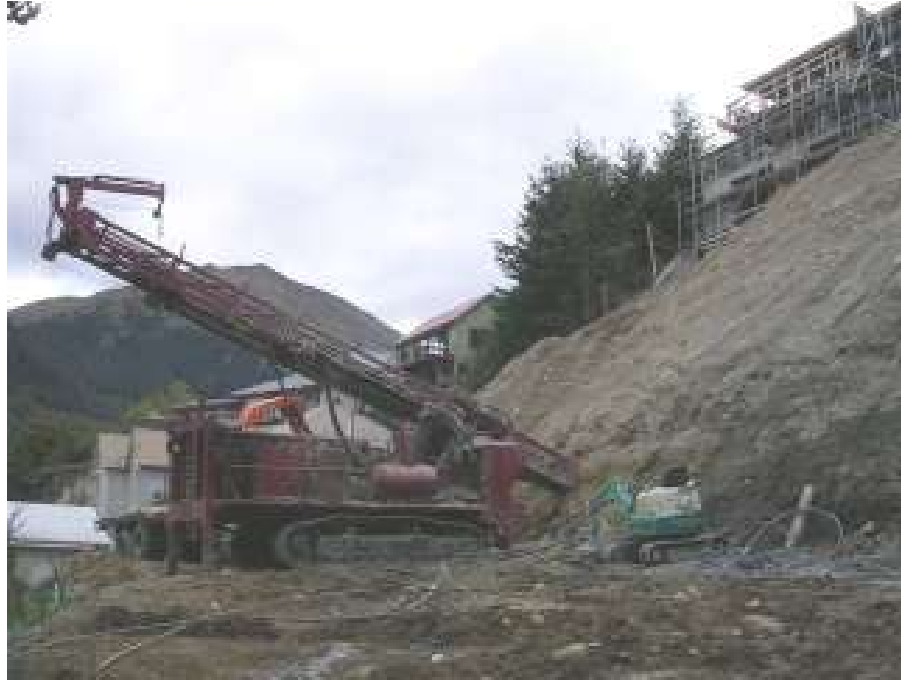
Plate 1 Rig installing trial nails before excavation provides an 80° soil nailed face.
