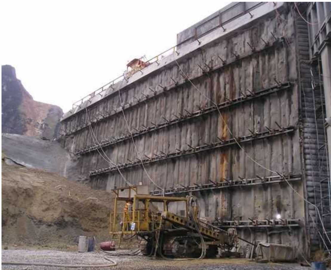
Photo 1 Freeport Mine Anchored piled wall to Crusher 6 Dump Slab
