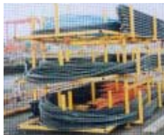
SBMA anchor tendons are double corrosion protected.
