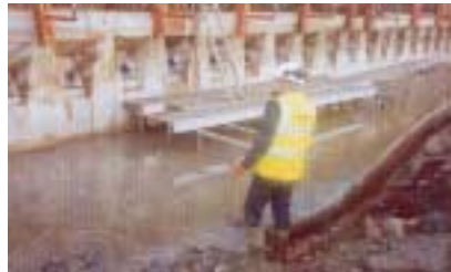
Capping beam with anchor installation nearly complete.
