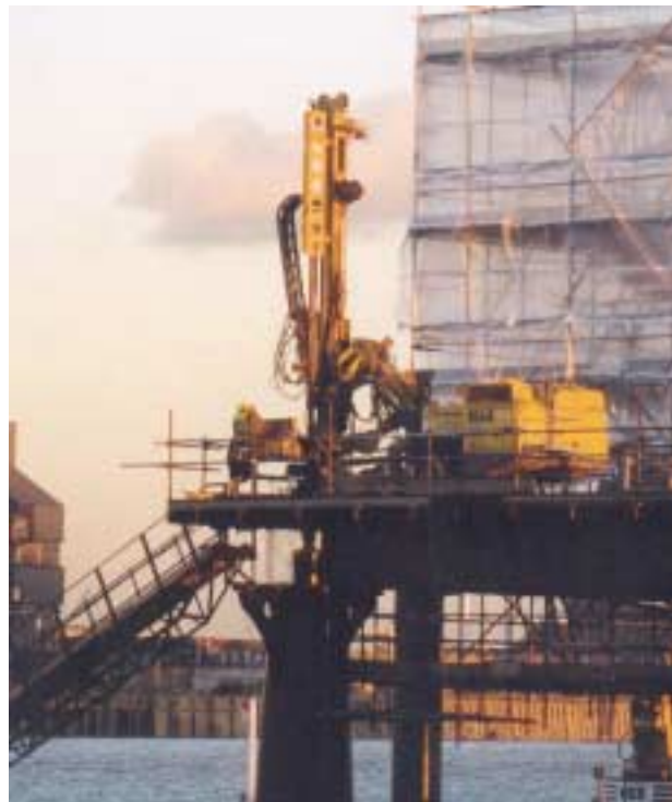
Photo 2. Casagrande drill rig.
