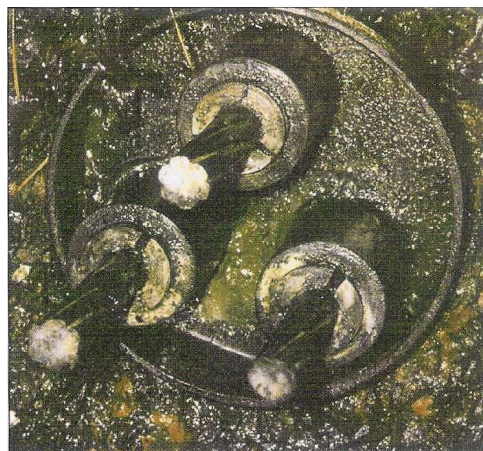
Photograph 2. Shows benefits when using grease filled protection caps.
