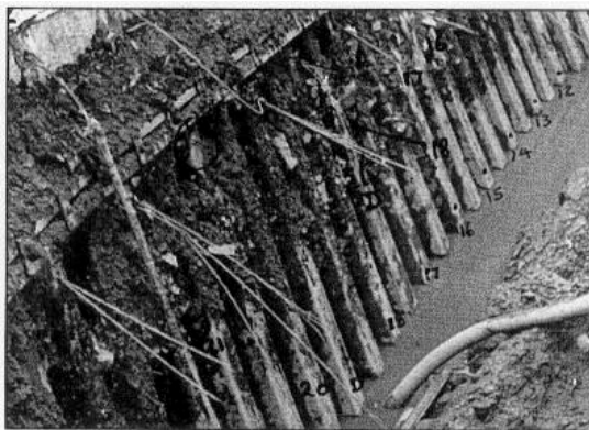
Photo 3: Severed anchor tendons after wall failure
