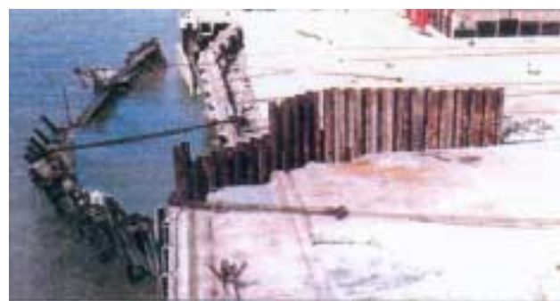
Photo 2: Overall view of wall failure after about 2 weeks (left)
